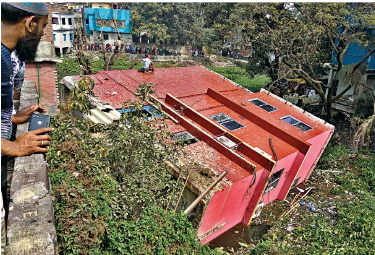
A three-storey building lying on its side after it toppled in Keraniganj's Charail Khelarmath area yesterday morning. Members of the fire service rescued eight people -- seven of them injured -- from the building. Officials said it might have collapsed due to faulty construction.
