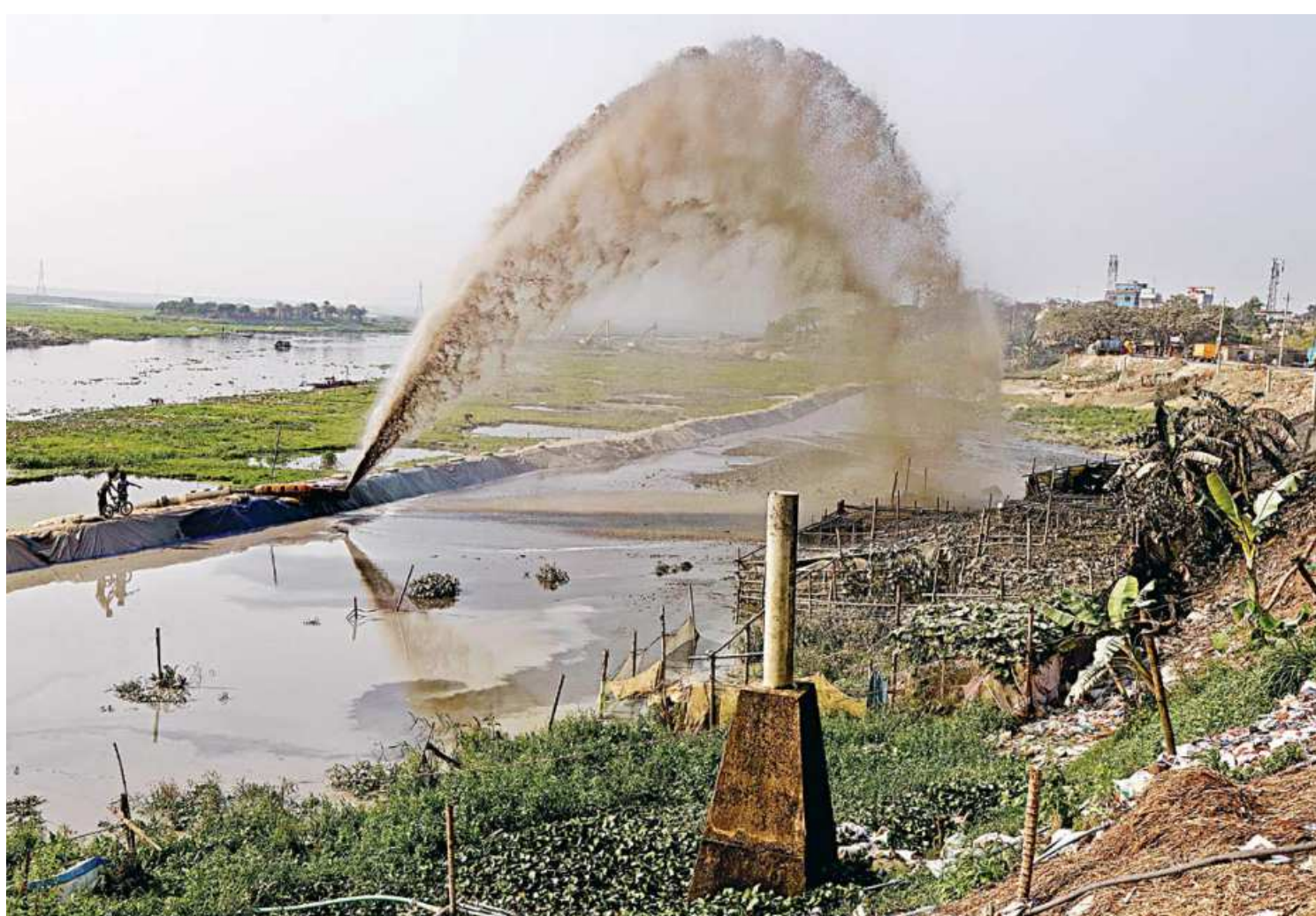
Dredging of the Turag river going on in the capital’s Mirpur Beribadh to increase the navigability of the river, which bears a dried-up appearance. The photo was taken yesterday.
