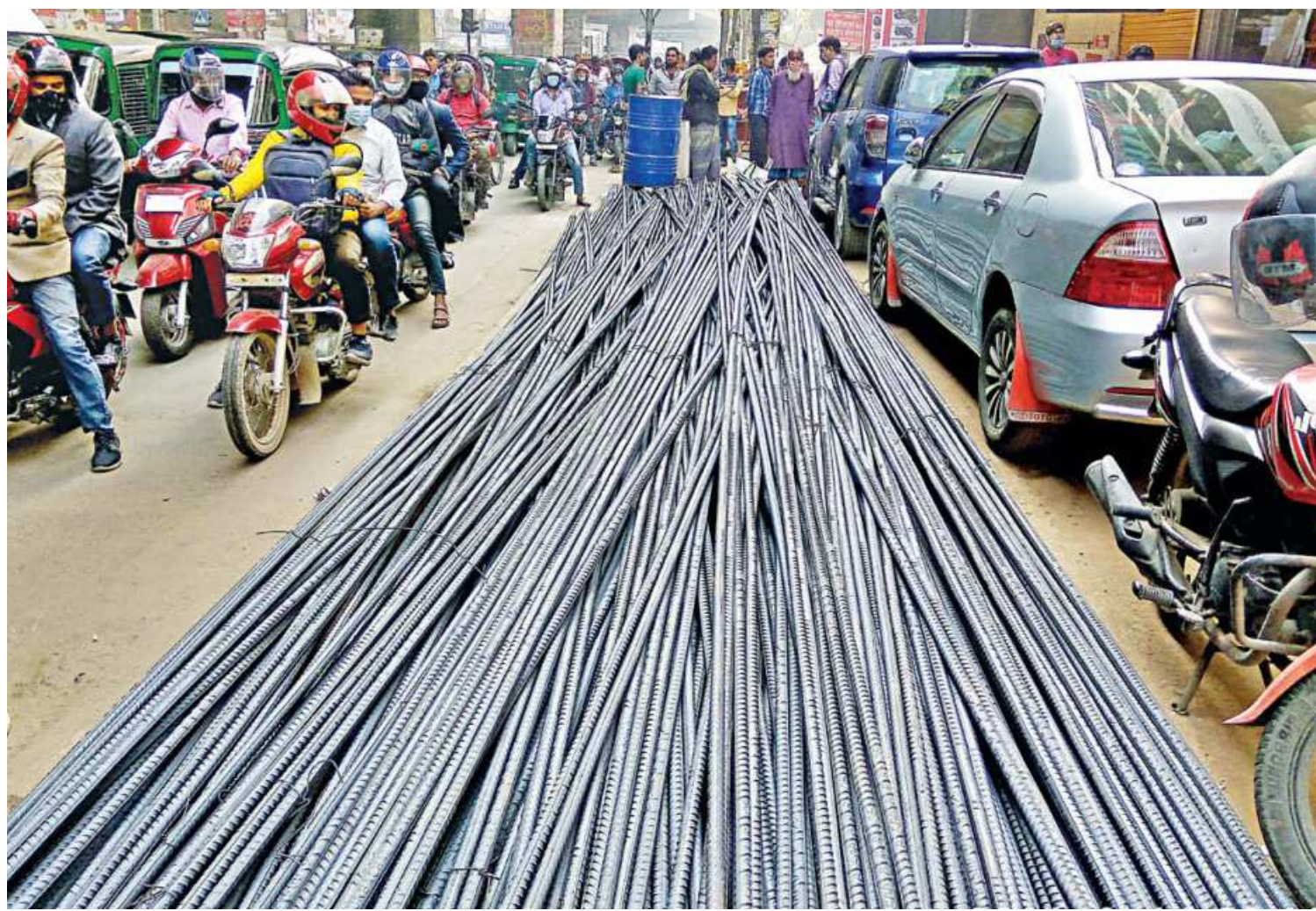
Iron rods for a building under construction occupy a part of the road while vehicles are illegally parked on the pavement, putting pedestrians' and motorists' lives in danger on Tongi Diversion Road in the capital's Moghbazar area. The photo was taken yesterday.
