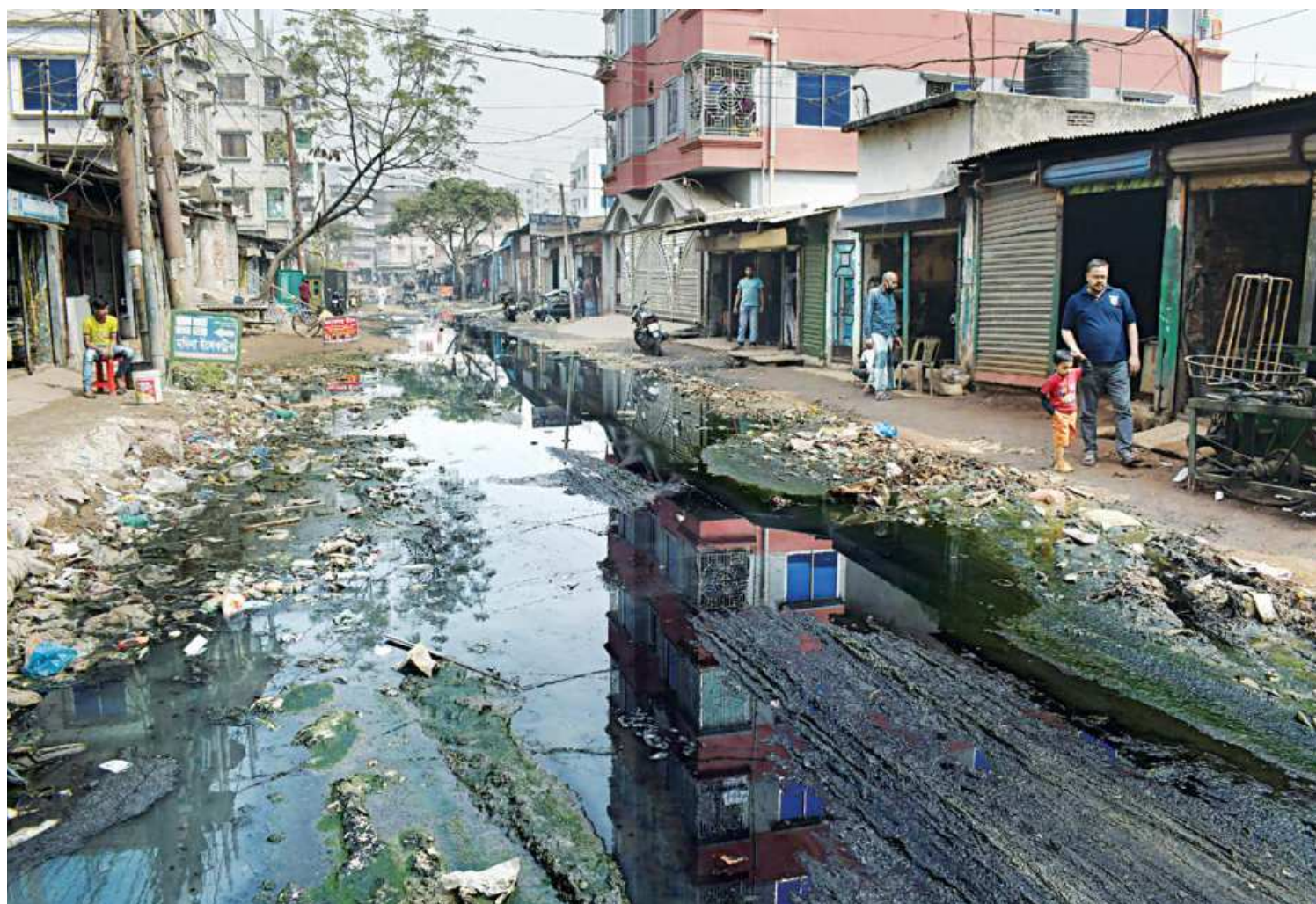
Filthy water from nearby dyeing factories and sewage stagnated on Shyampur-Kadamtoli street in the capital due to poor drainage system. Almost the entire street has become unusable. Pedestrians in Rajuk residential area in Shyampur suffer the most as they have to endure the stench. The photo was taken yesterday.
