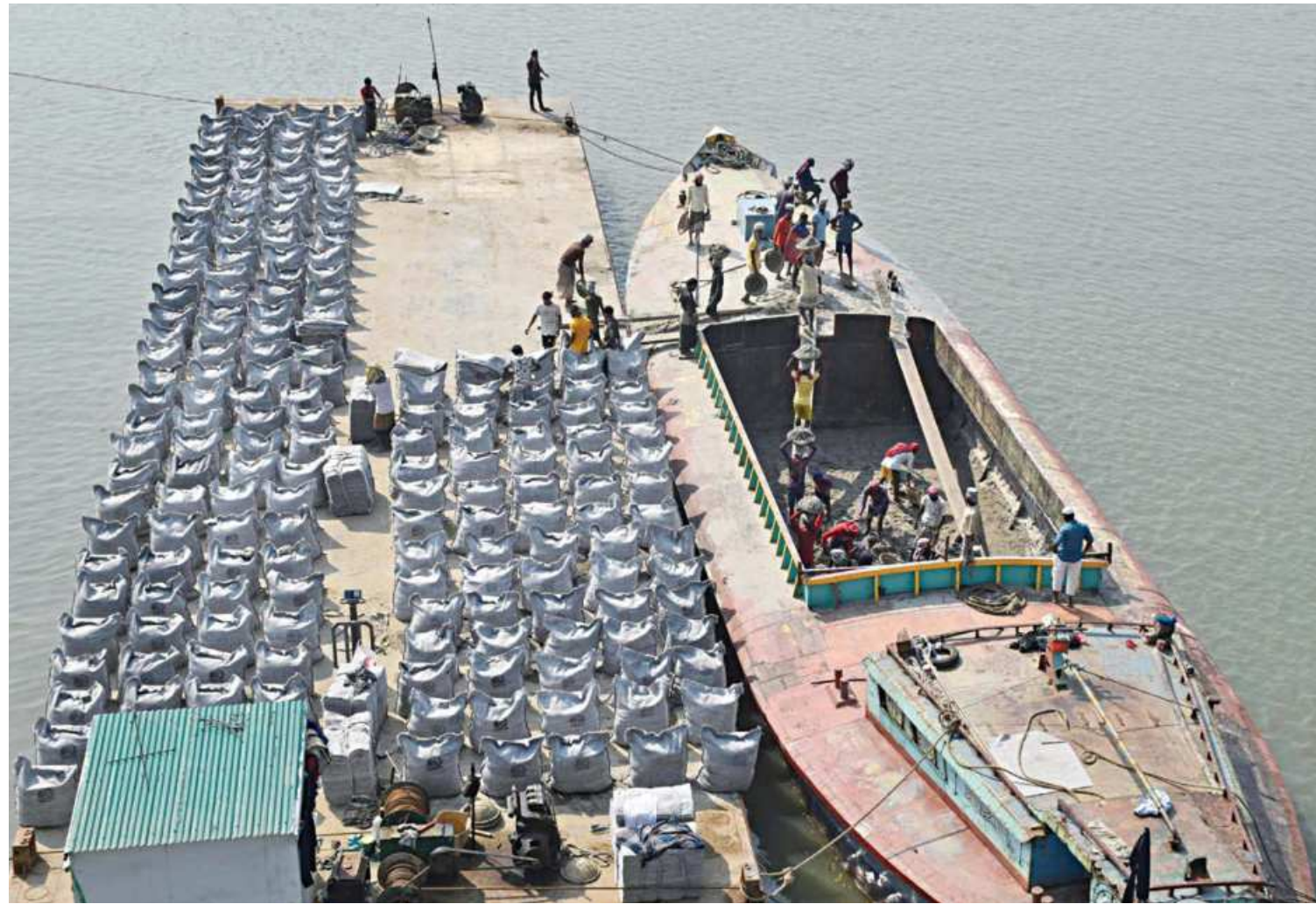
The Bangladesh Water Development Board is using a barge as a platform for preparing sandbags. A bulk carrier has brought in the sand. The bags would be dumped in different spots along the Sugandha river of Barishal's Babuganj upazila where erosion is severe. The photo was taken from Doarika area recently.
