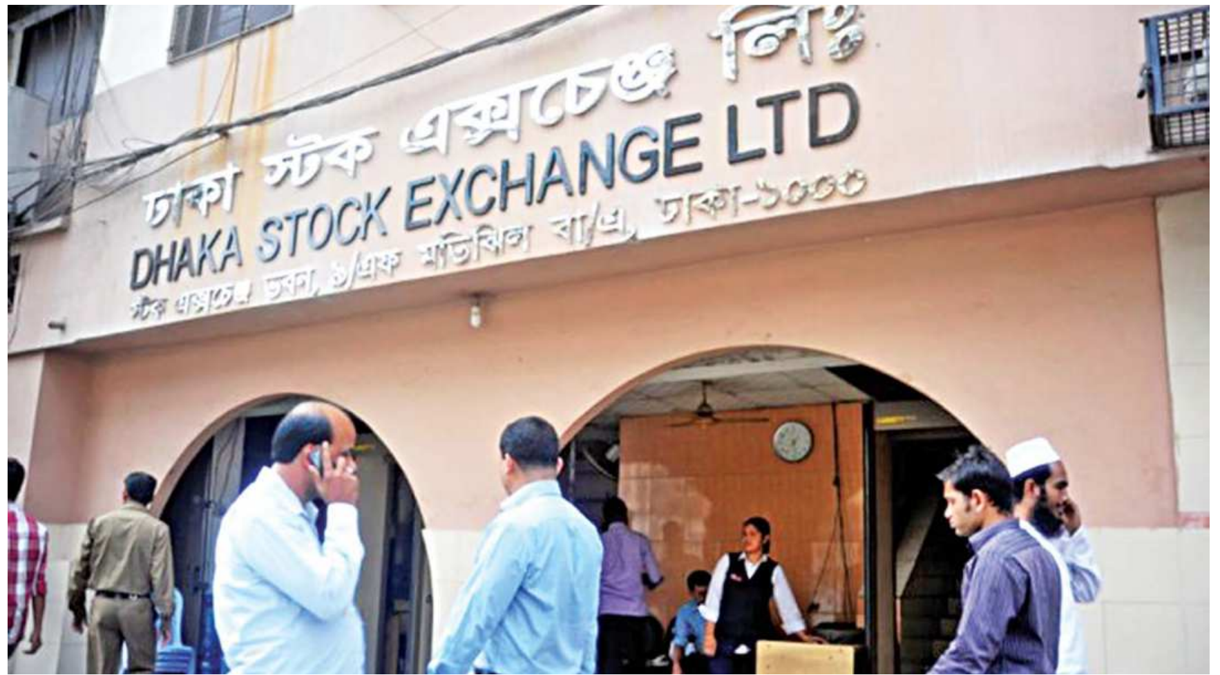
The Dhaka Stock Exchange building.
