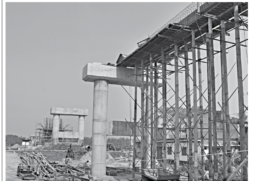
The current state of the under construction bridge on the Lohalia river near Patuakhali town.
