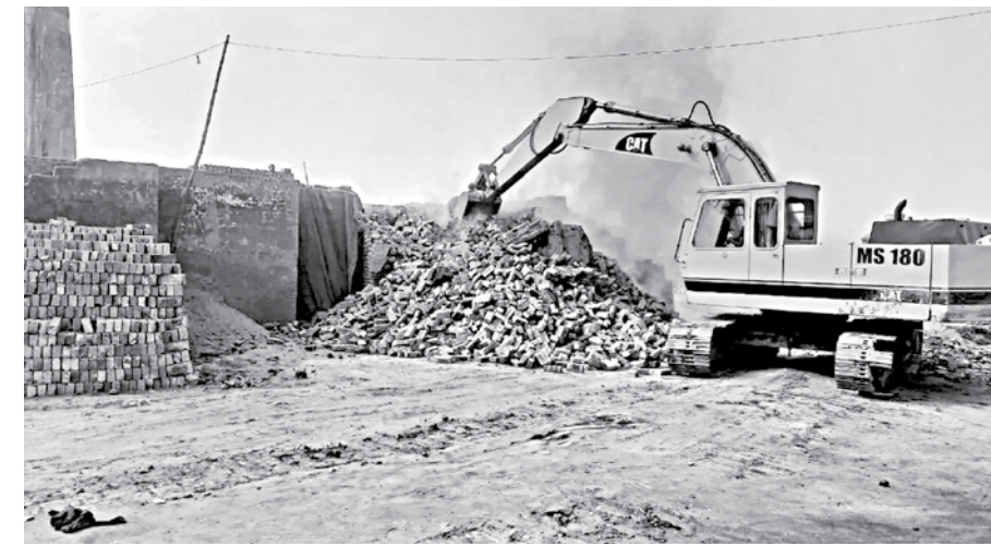
An illegal brick kiln being demolished in Savar as part of the Department of Environment's daylong drive yesterday.
