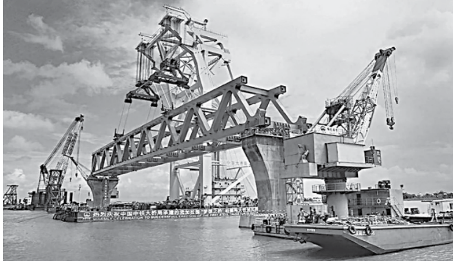
Ongoing construction works of the Padma Bridge, one of the major infrastructural development projects initiated by Bangladesh.
