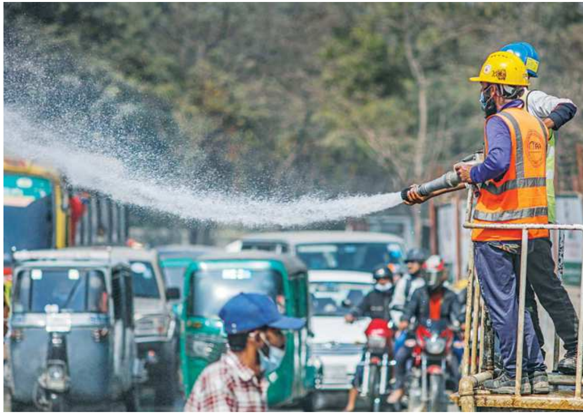
Workers of Dhaka Mass Rapid Transit Development Project hose the road in the capital's Khamarbari area, to suppress the dust that is produced due to the construction of the metro rail lines. Air quality in the capital often gets to hazardous level in winter, owing to dry weather. The photo was taken yesterday.
