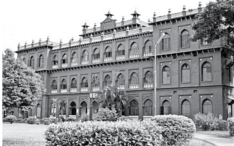
The Curzon Hall building in Dhaka University.
