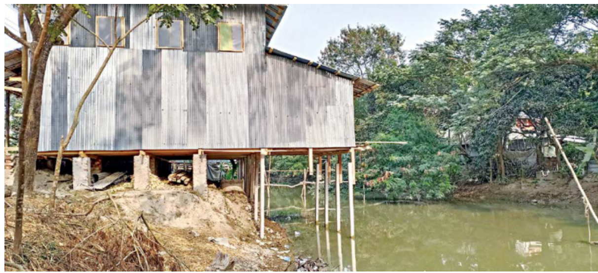
Illegal structures are being built on the canal in Kalapara upazila of Patuakhali.
