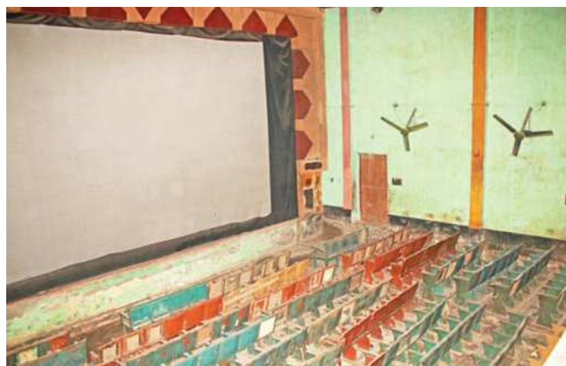
A desolate Sikta Cinema Hall Private Limited awaits demolition after operating for 28 years.
