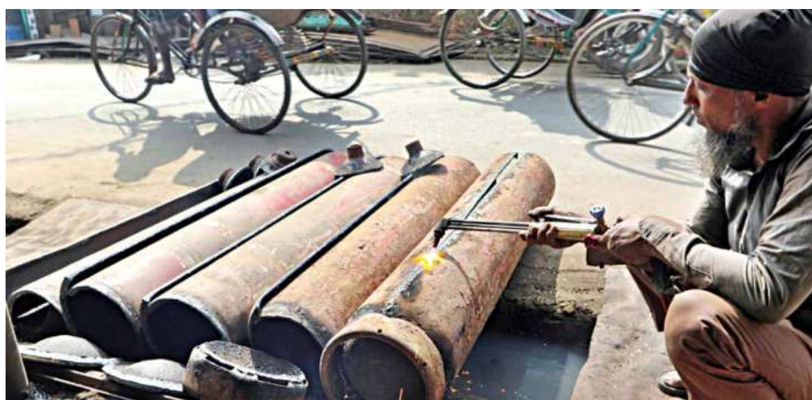
A man cutting scrap, collected from ship-breaking yards, with a blow torch and without maintaining any safety measures on a footpath in Chattogram. The oxygen cylinders, once used in ships, are turn into kitchen tools that have a huge demand in the local market. The photo was captured from Ashraf Ali Road in the port city.
