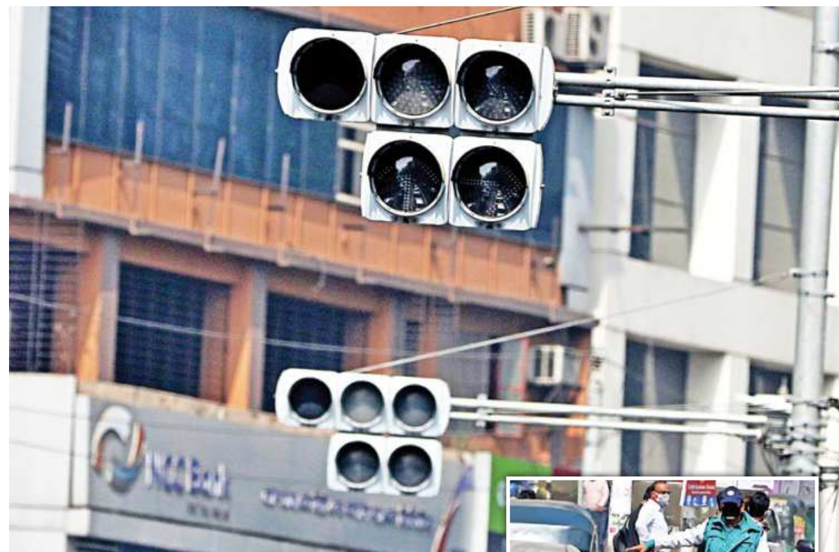
Traffic lights at Gulshan-1, a major intersection in one of the most upscale neighbourhoods of the capital, remain out of order, as traffic police are left with the task to manage the busy thoroughfare with hand signals, inset. The photos were taken yesterday.
