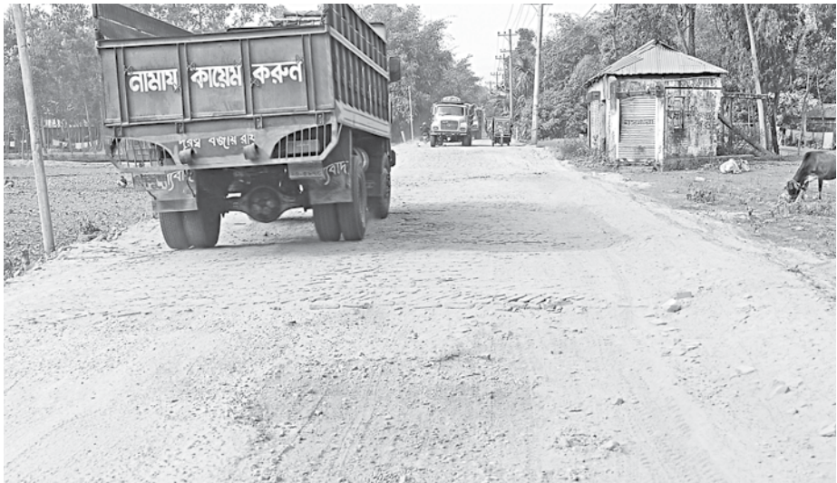
The inner brick layer has been exposed after the asphalt layer on top was damaged in a large section of the 100-kilometre-long highway that connects Lalmonirhat with Burimari land port. The unpredictable road, also riddled with huge potholes, has been causing frequent accidents for a long time.
