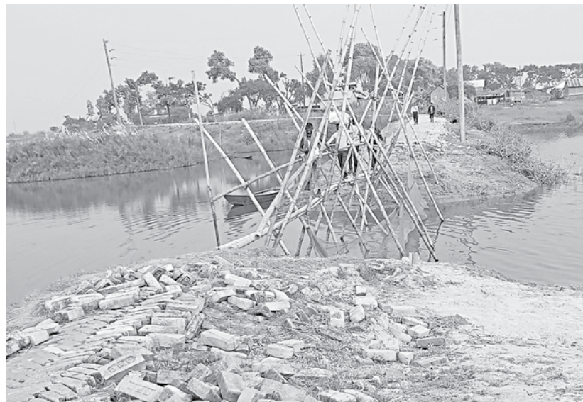
Locals use the temporary bamboo bridge on a canal in Char Jhaukanda union in Faridpur's Charbhadrasan upazila amid risk of accident.
