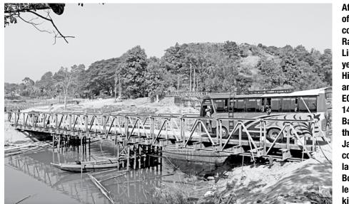
After nearly two weeks of suspension road communication through Rangamati-Khagrachhari Link Road resumes yesterday. The Roads and **Highways Department** and Bangladesh Army 20 ECB jointly constructed a 140-feet-long temporary Bailey bridge next to the collapsed one. On January 12, the bridge collapsed when a stoneladen truck was crossing Boro Mohapurom Chhara, leaving three peoples killed. PHOTO: STAR 1186 41: 51.05.0000.001.22.002.52**-00**2
