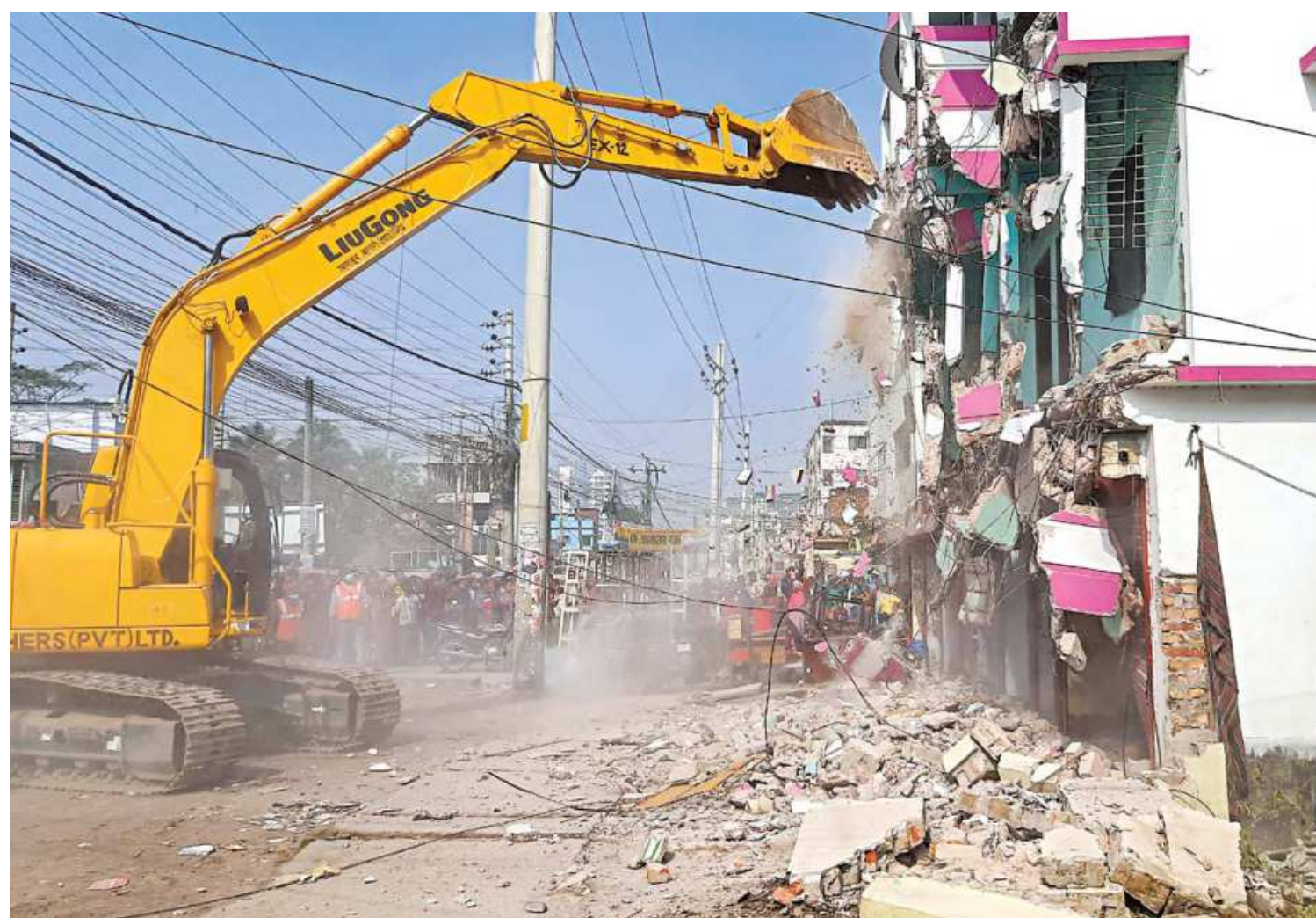
Roads and Highways Department has been demolishing illegal structures on Khulna city's Sher-e-Bangla Road for a week, to turn the two-lane road into a four-lane one. Till yesterday, around 70 buildings were demolished during the ongoing eviction drive. The photo was taken from Amtola intersection yesterday.
