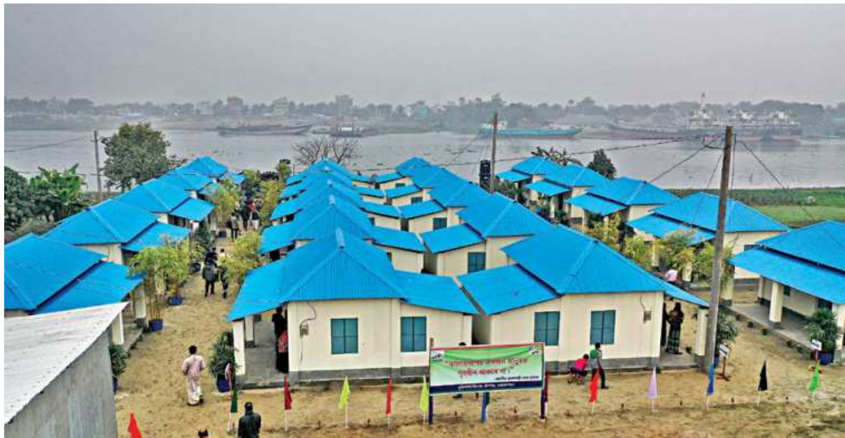
A view of a cluster of houses in Rugganj's Murapara area, built under the Ashrayan-2 project. The government is building such houses for landless and homeless families to mark Mujib Borsho. Prime Minister Sheikh Hasina will inaugurate the virtual handover ceremony today. The photo was taken on Thursday. PHOTO: ANISUR RAHMAN
