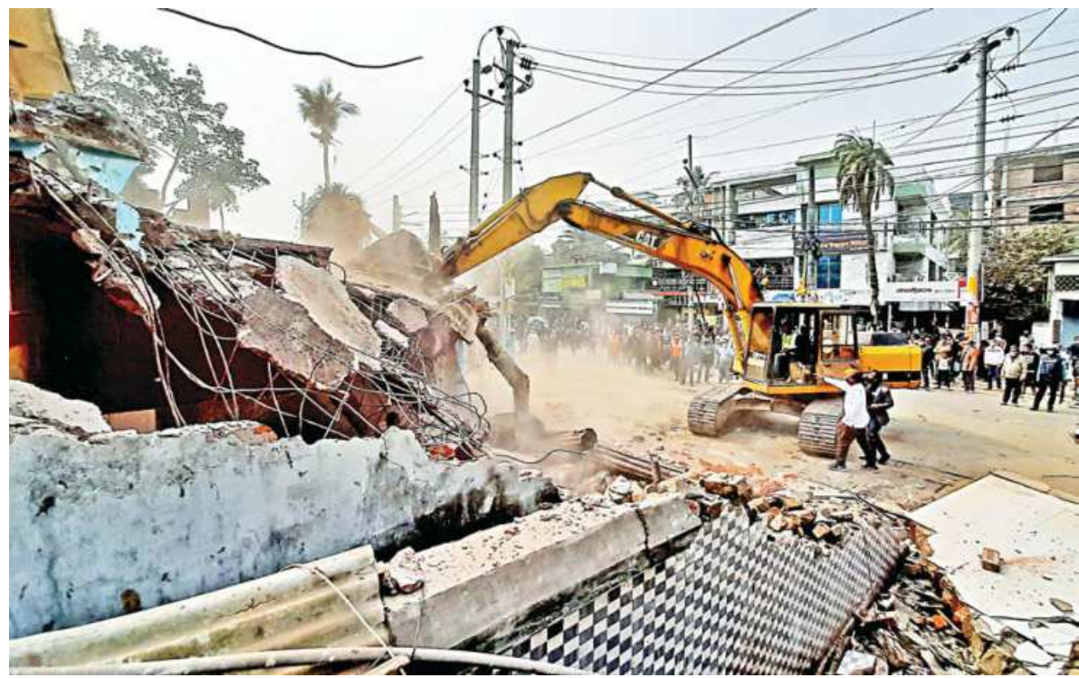
An excavator demolishing a structure in Khulna's Moylapota area. The roads and highway department, with assistance from the Khulna City Corporation, conducted the drive to demolish structures that had encroached upon the road, which will be turned into a four-lane highway. The photo was taken around 11:30am yesterday.
