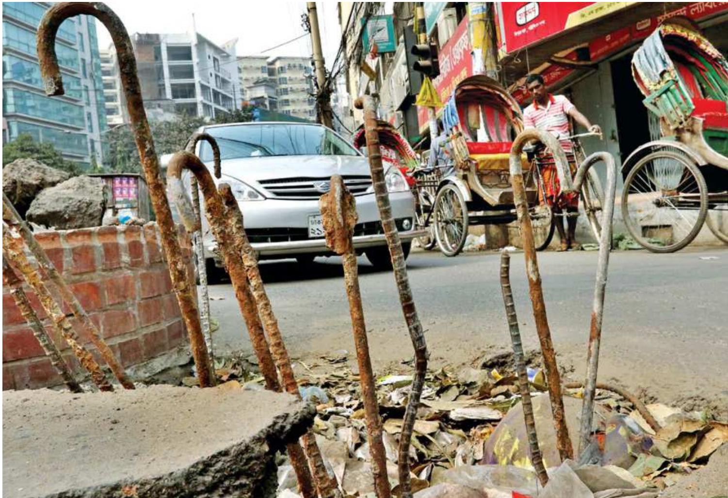
Rods sticking out of a manhole on the side of a road at the north-west corner of the Panthapath intersection in the capital. According to locals, the cover of the manhole had broken around a month ago and people had bent its rods outward to ward off vehicles. However, contrary to that purpose, the rods pose a danger to vehicles which pass perilously close. The photo was taken recently.
