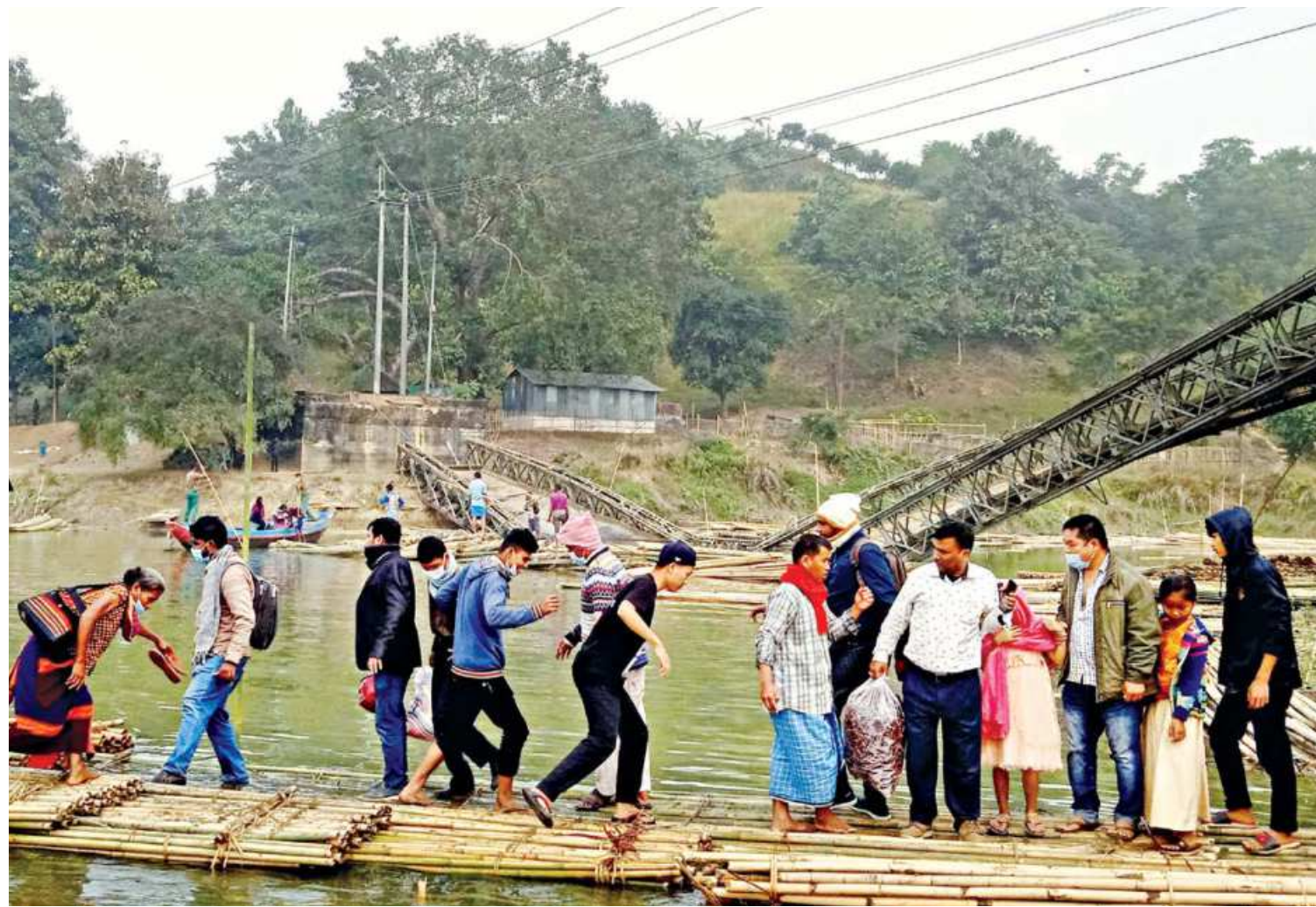
People using a "bridge" made of bamboo that was being transported on the Boro Mohapuro river in Khagrachhari Sadar upazila as a bailey bridge behind them collapsed around 6:30am yesterday, unable to take the load of a stone-laden truck. Road communication between Khagrachhari and Rangamati was severed and three people were killed.
