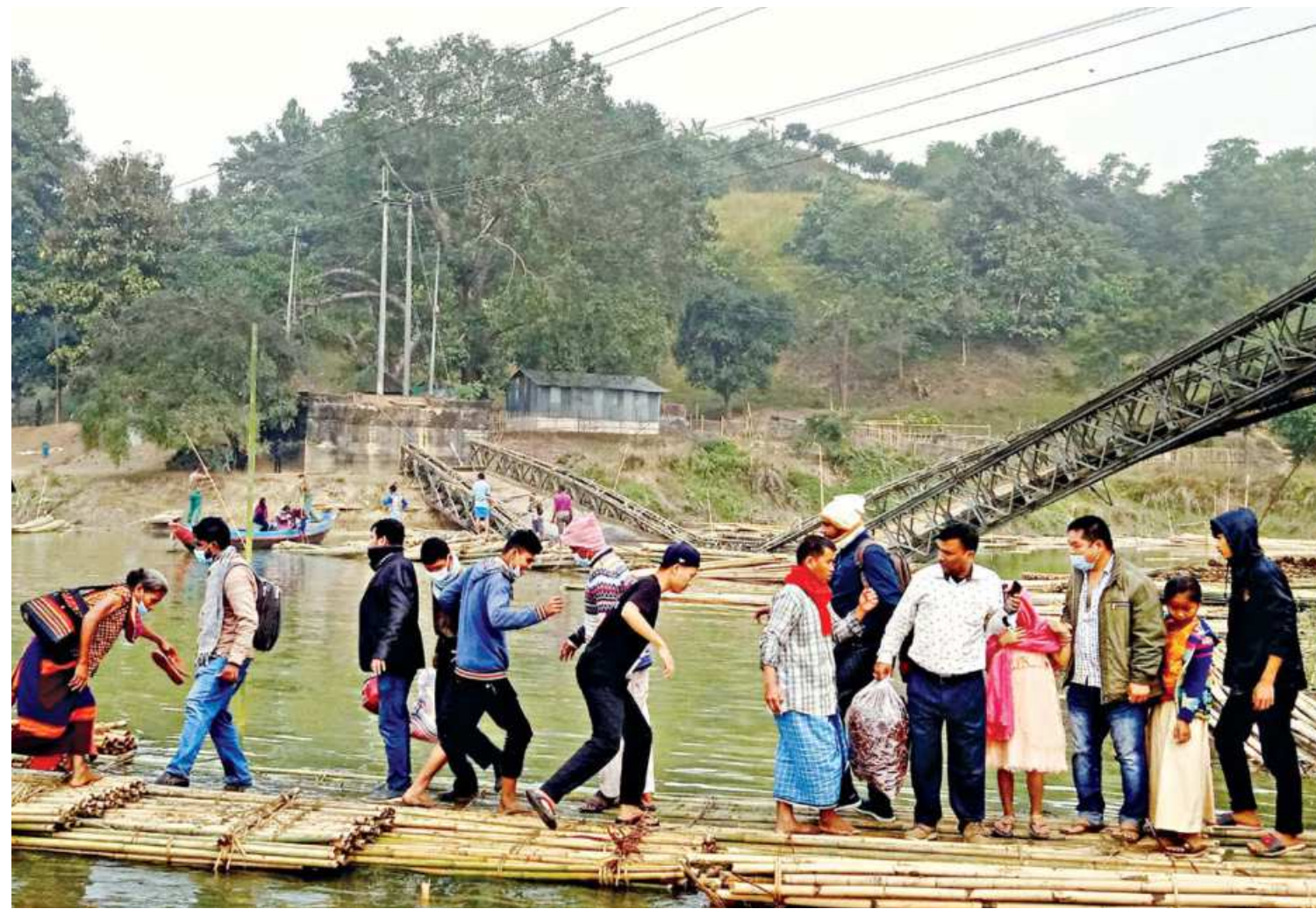
People using a "bridge" made of bamboo that was being transported over the Boro Mohapuro river in Khagrachhari Sadar upazila as a bailey bridge behind them collapsed around 6:30am yesterday unable to take the load of a stone-laden truck. Road communication between Khagrachhari and Rangamati was severed and three people were killed.
