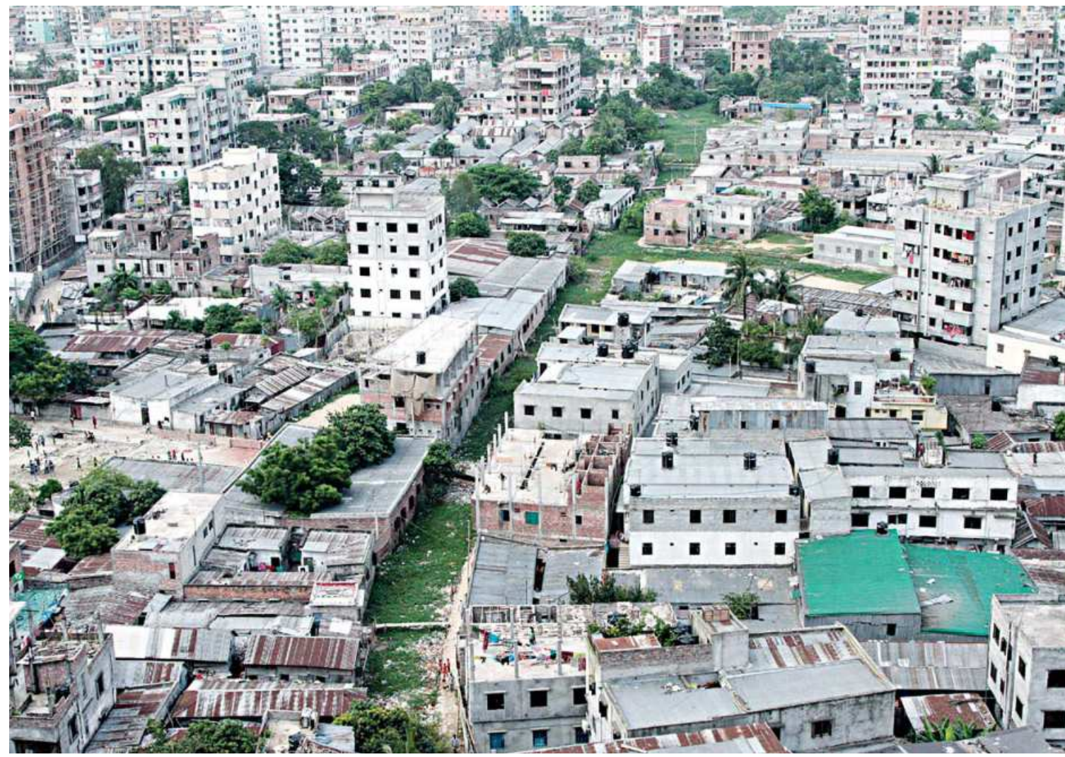
This photo taken a few years ago shows Shazadpur Canal at Badda in the capital completely clogged by garbage and vegetation. Such canals under the DNCC could be revived soon.
