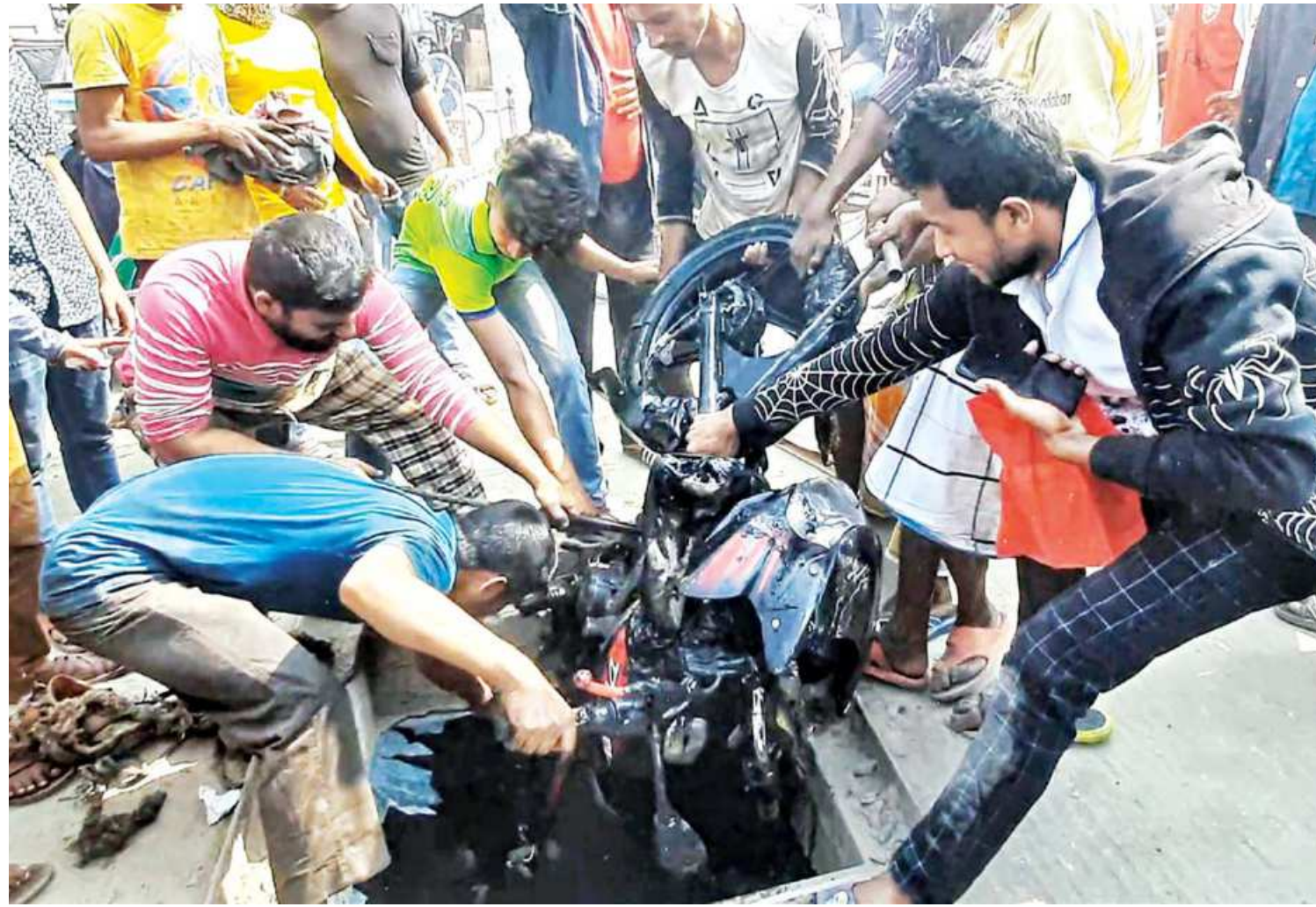
A motorcycle being pulled out of a manhole on KDA Avenue in Khulna city after a biker fell into it yesterday. The accident happened as the authorities concerned removed the cover for work in sewerage lines on both sides of the road.
