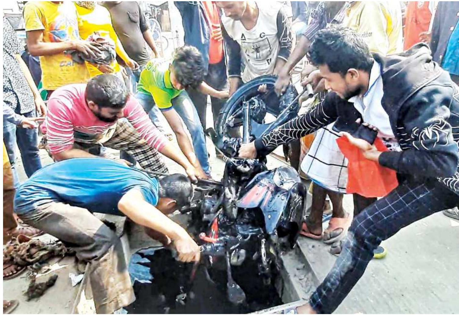
A motorcycle being pulled out of a manhole on KDA Avenue in Khulna city after a biker fell into it yesterday. The accident happened as the authorities concerned removed the cover for work in sewerage lines on both sides of the road.
