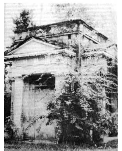
The Greek monument in Dhaka before the repair
