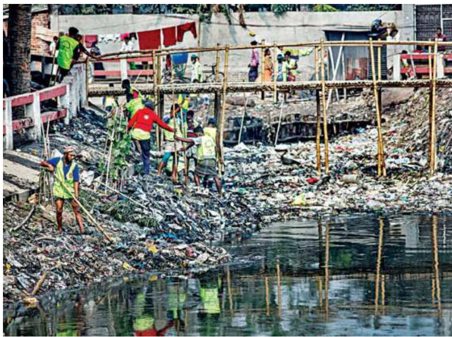
Workers of Dhaka North City Corporation cleaning Ramchandrapur canal in the capital's Adabor area yesterday. The responsibility to maintain the canal was recently shifted to the corporation from the Dhaka Water Supply And Sewerage Authority.
