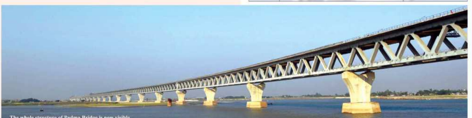
The whole structure of Padma Bridge is now visible
