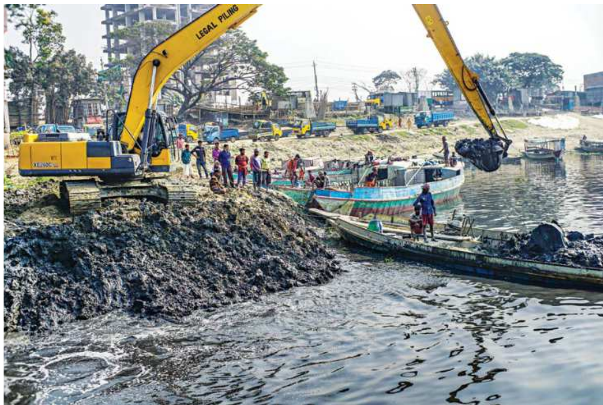
Workers of the BIWTA excavating sediment to increase the navigability of the Turag river in and around its Mirpur's Diabari landing station yesterday. The soil is later sold.
