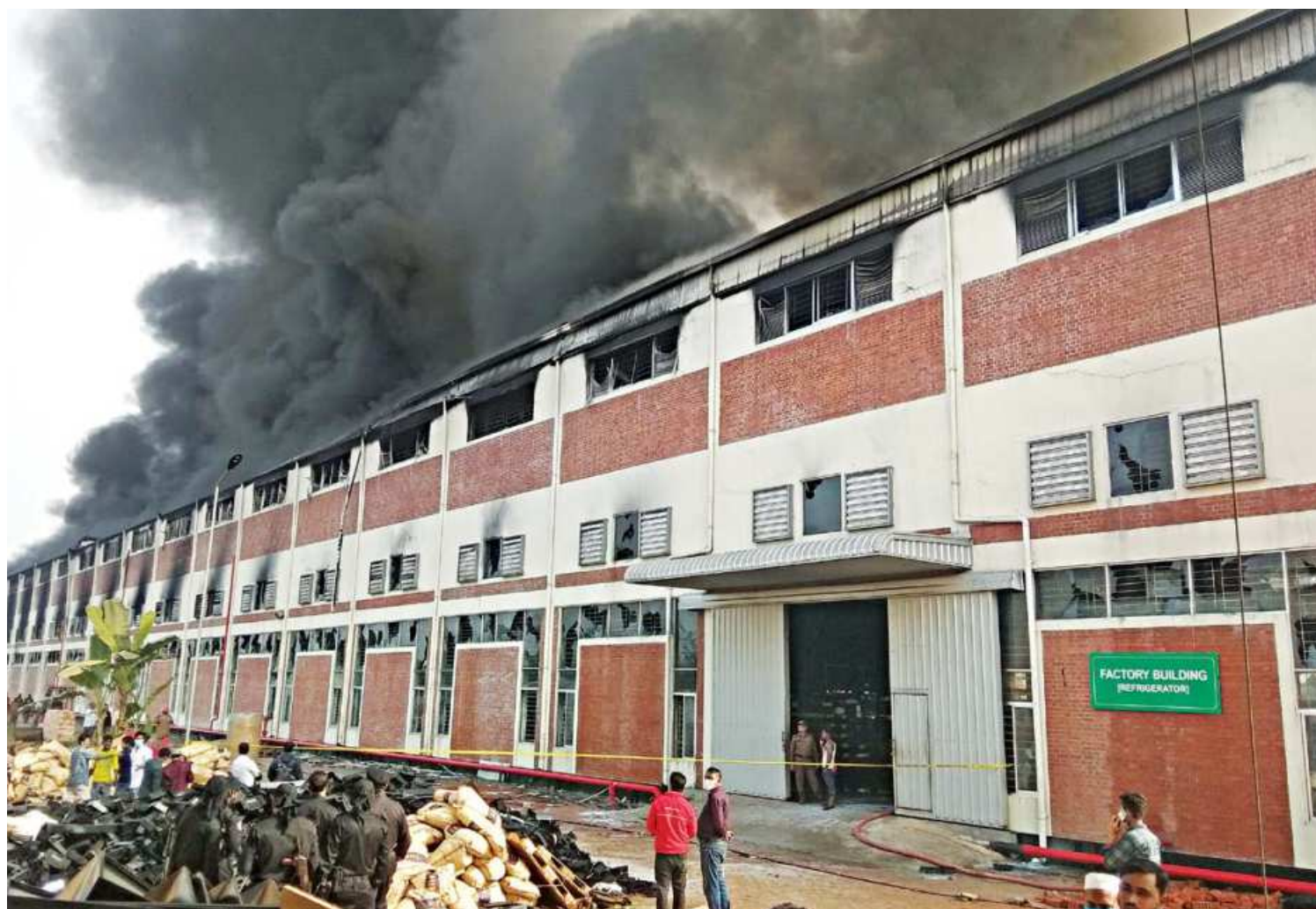
The factory of Konka refrigerators in Narayanganj's Sonargaon upazila caught fire around 11:00am yesterday. Thirteen fire engines doused the fire after almost two-and-a-half hours of work. One engineer of the factory was injured as he tried to escape the fire by jumping off the building.
