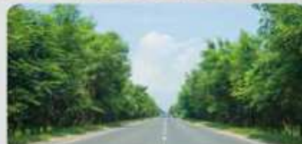
Kushtia Bypass Road
