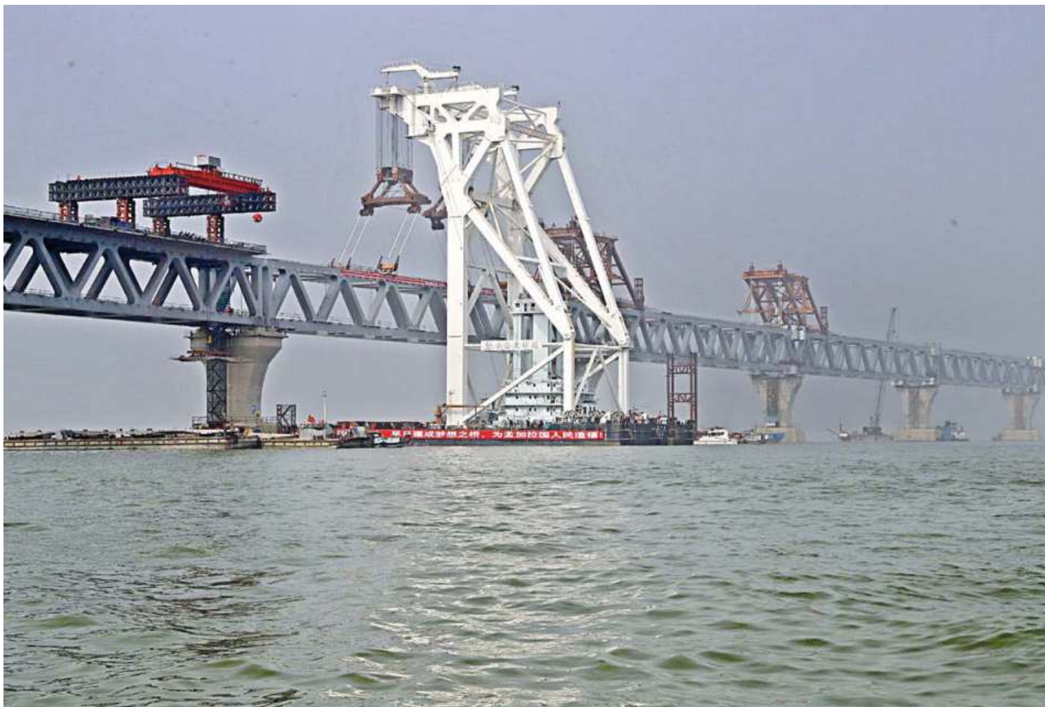
A gigantic floating crane finishes installing the last span, measuring 150 metres, on pillars 12 and 13 of the Padma bridge around noon yesterday. The entirety of the 6.15-km long bridge is now visible, bringing hopes of connecting the country's 21 south-western districts to the capital closer to fruition.
