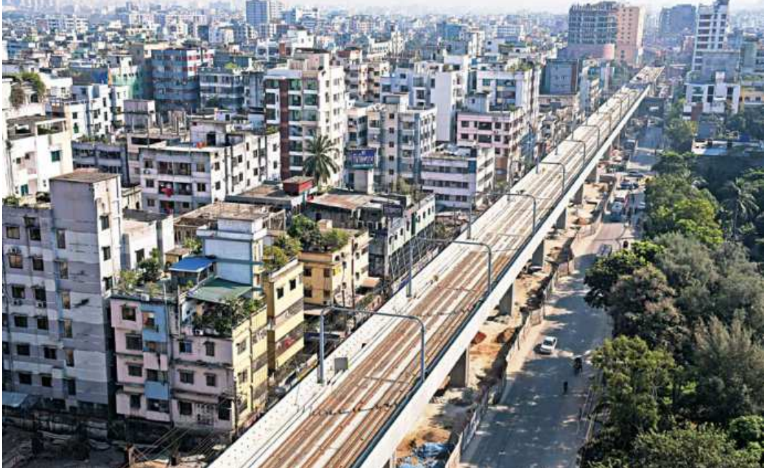
A portion of the metro rail project is seen in Mirpur, Dhaka. The photo was taken last week.
