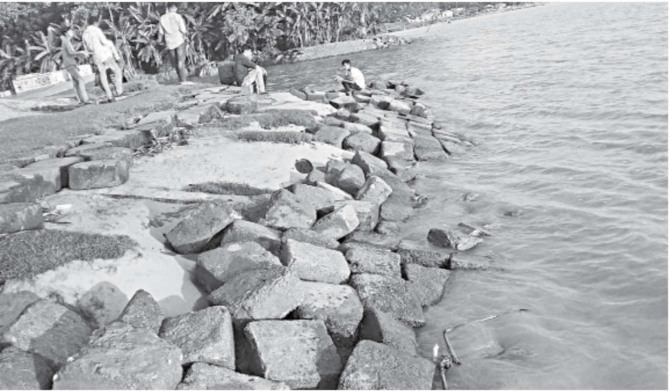
The concrete blocks of the dyke on the bank of the Payra river in Barguna's Amtali upazila town have been washed away, threatening the town.
