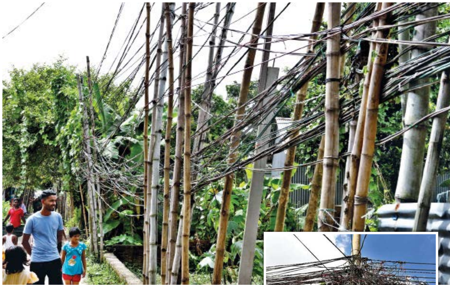
Electricity connections to many houses in Norsinhgpur area of Narayanganj's Fatulla have been set up using bamboo poles. Such connections put the power users and locals at risk of accidents. Locals say they are forced to use bamboo poles as the concrete ones, installed by the authorities, are far apart from each other. Inset, a tangled mess of wires on a pole in the area. The photos were taken yesterday.
