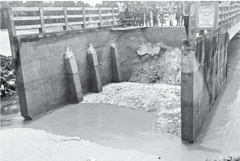
Strong current washed away a portion of the approach road on the eastern side of Boro Basalia bridge on the Louhajang river in Tangail Sadar upazila on Sunday morning, causing suspension of road communication in the area.
