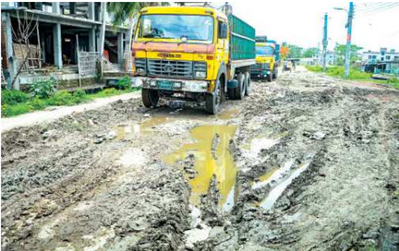
Bituminous surface has totally disappeared from Bastuhara bypass road in Khulna. The photo was taken recently.
