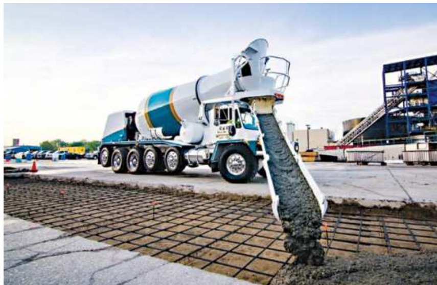
Discharging RMC through a chute
