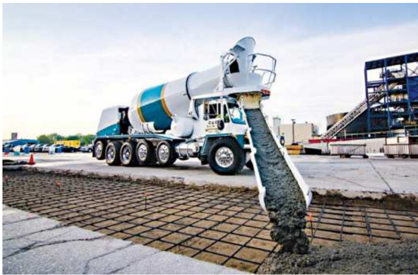
Discharging RMC through a chute
