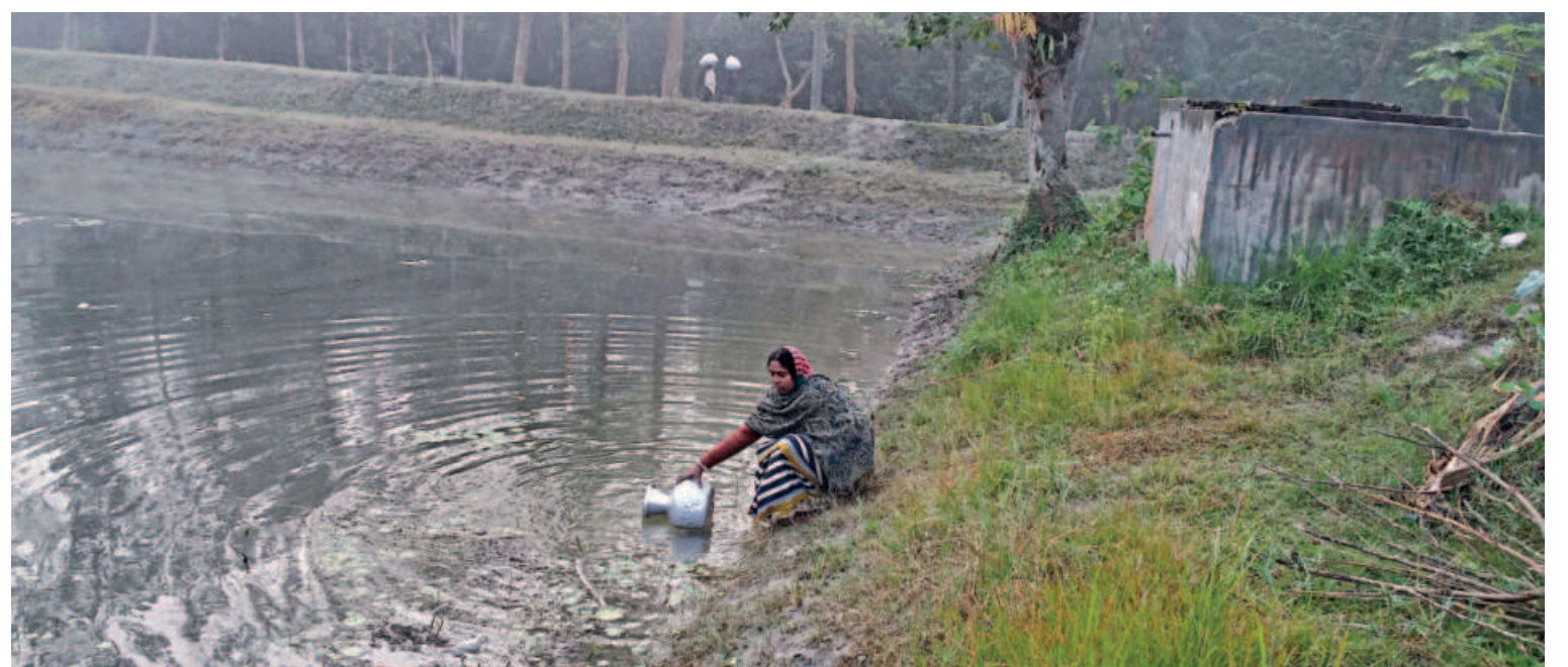
A woman collects water directly from a pond in Bagerhat's Sangdia village under Kachua upazila as pure drinking water is no longer available ever since the pond's sand filter, seen behind her, went out of order.
