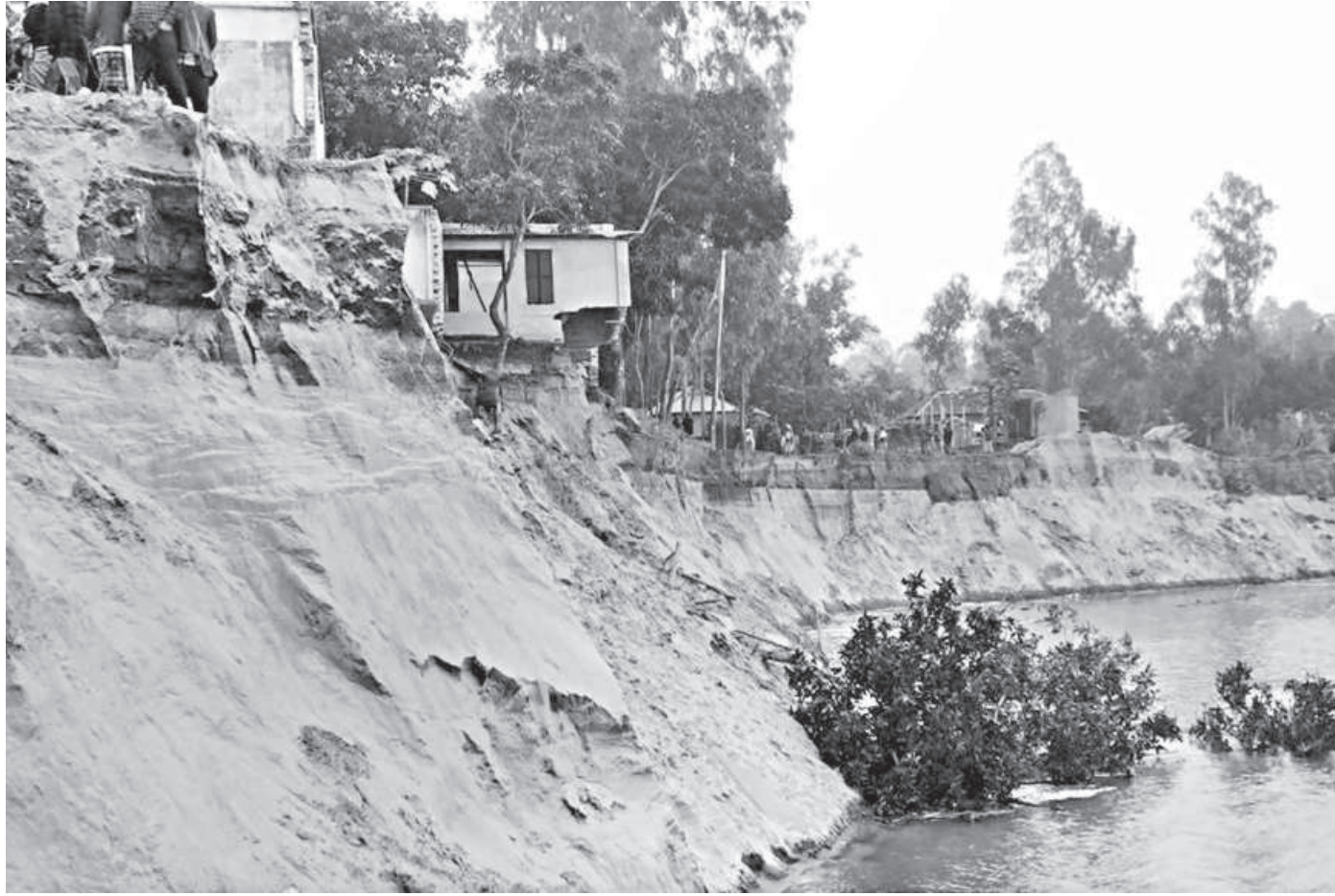
A part of the Jamuna river bank in Gorilabari village of Tangail's Kalihati upazila where at least five houses were destroyed by the river's erosion over the last three days and 10 more are under the risk of being destroyed. The photo was taken yesterday.
