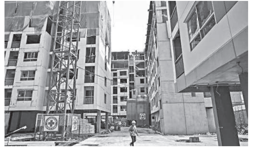
A worker walks in a construction site for buildings in Bangkok.
