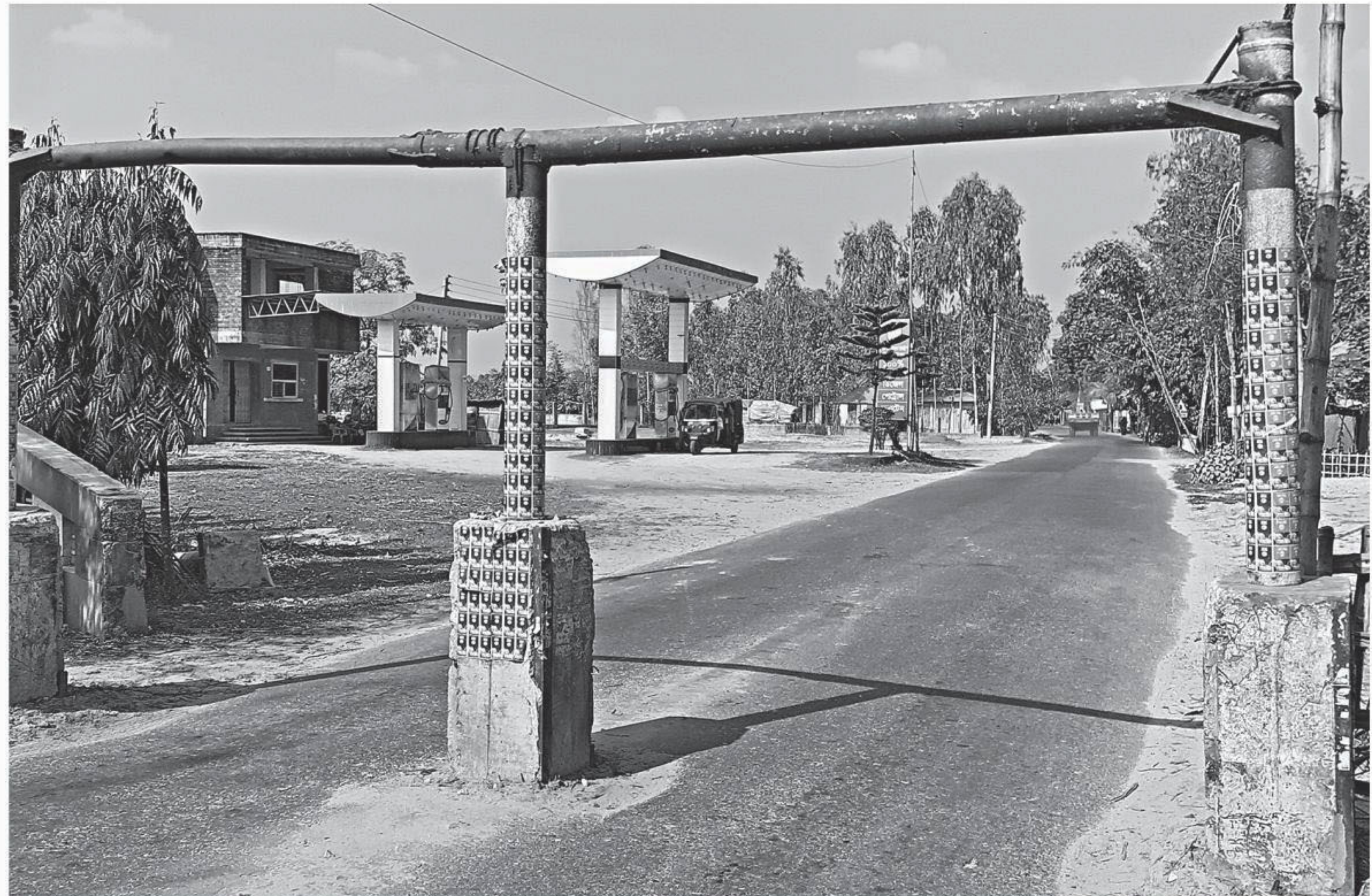
This barrier, set up by LGED on Kakina-Rangpur Road at the entrance of Sheikh Hasina Teesta Bridge after its inauguration in September last year, is still there, preventing plying of buses and trucks. PHOTO: S DILIP ROY
