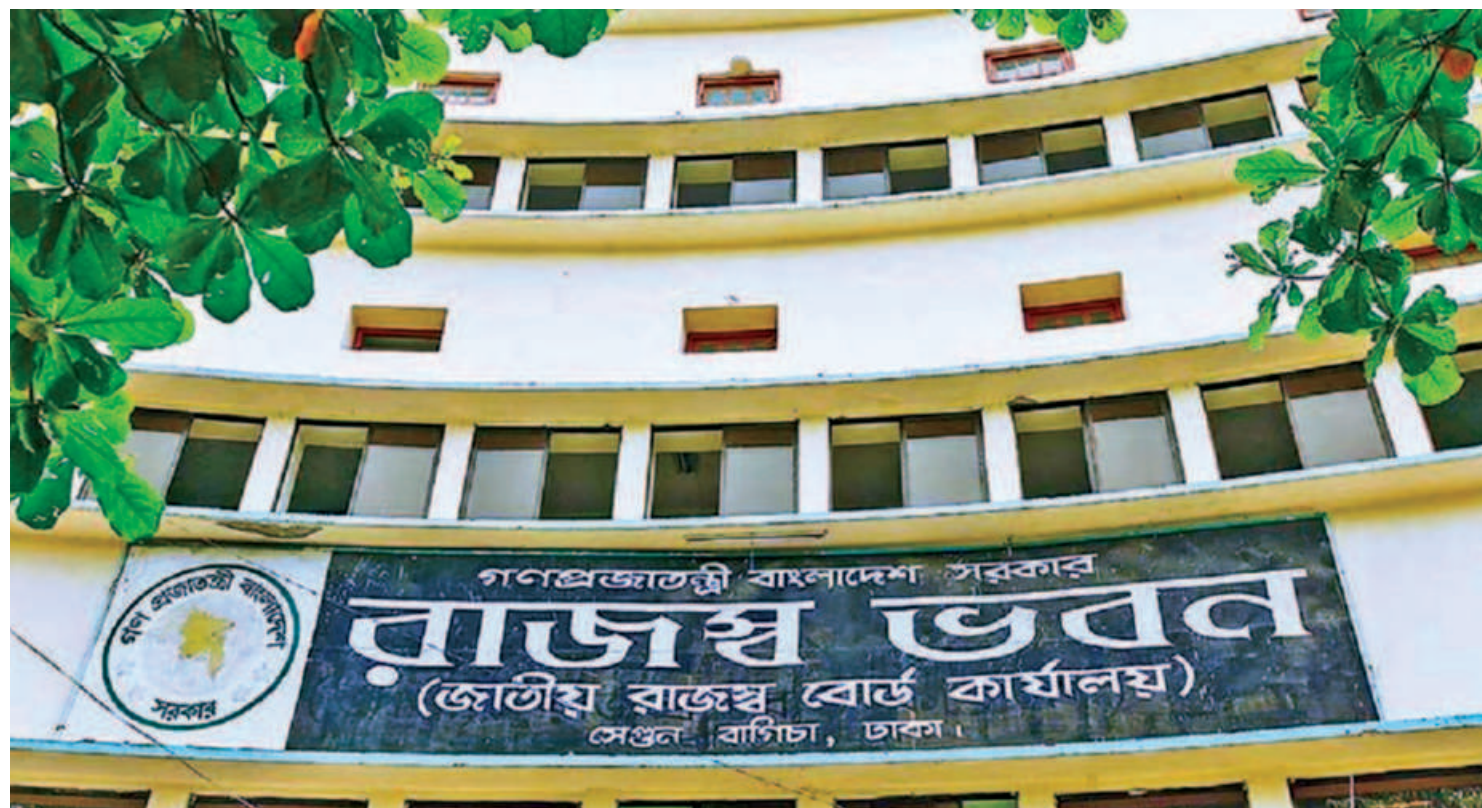
The headquarters building of the National Board of Revenue in Dhaka. Efficient taxation and fiscal policies can play a critical role in reducing inequalities and promoting inclusive sustainable development.
