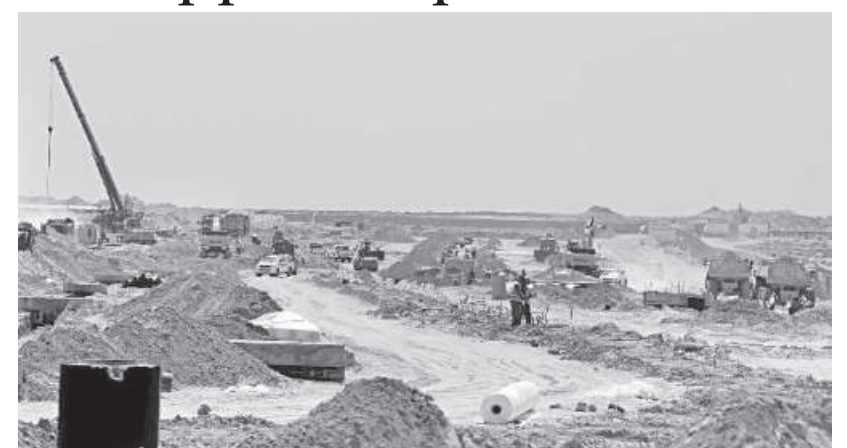
Labourers work at the construction site of Expo 2020 project in Dubai.
