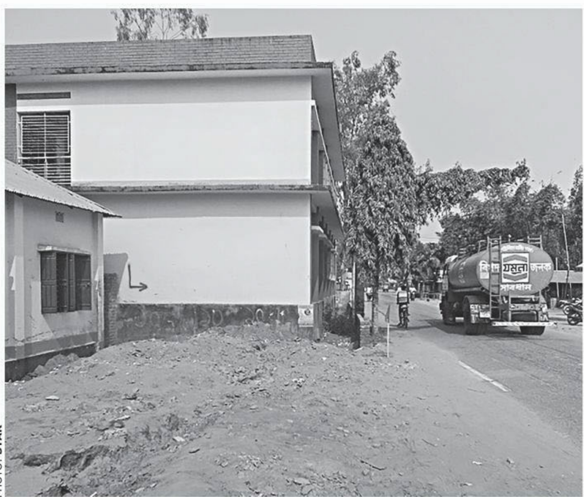
Local Government Engineering Department constructed the first floor of Dristinandan Government Primary School Nilphamari's Domar upazila in 2015 though Roads and Highways Department acquisitioned the school land (market in red arrow) in 2011.
