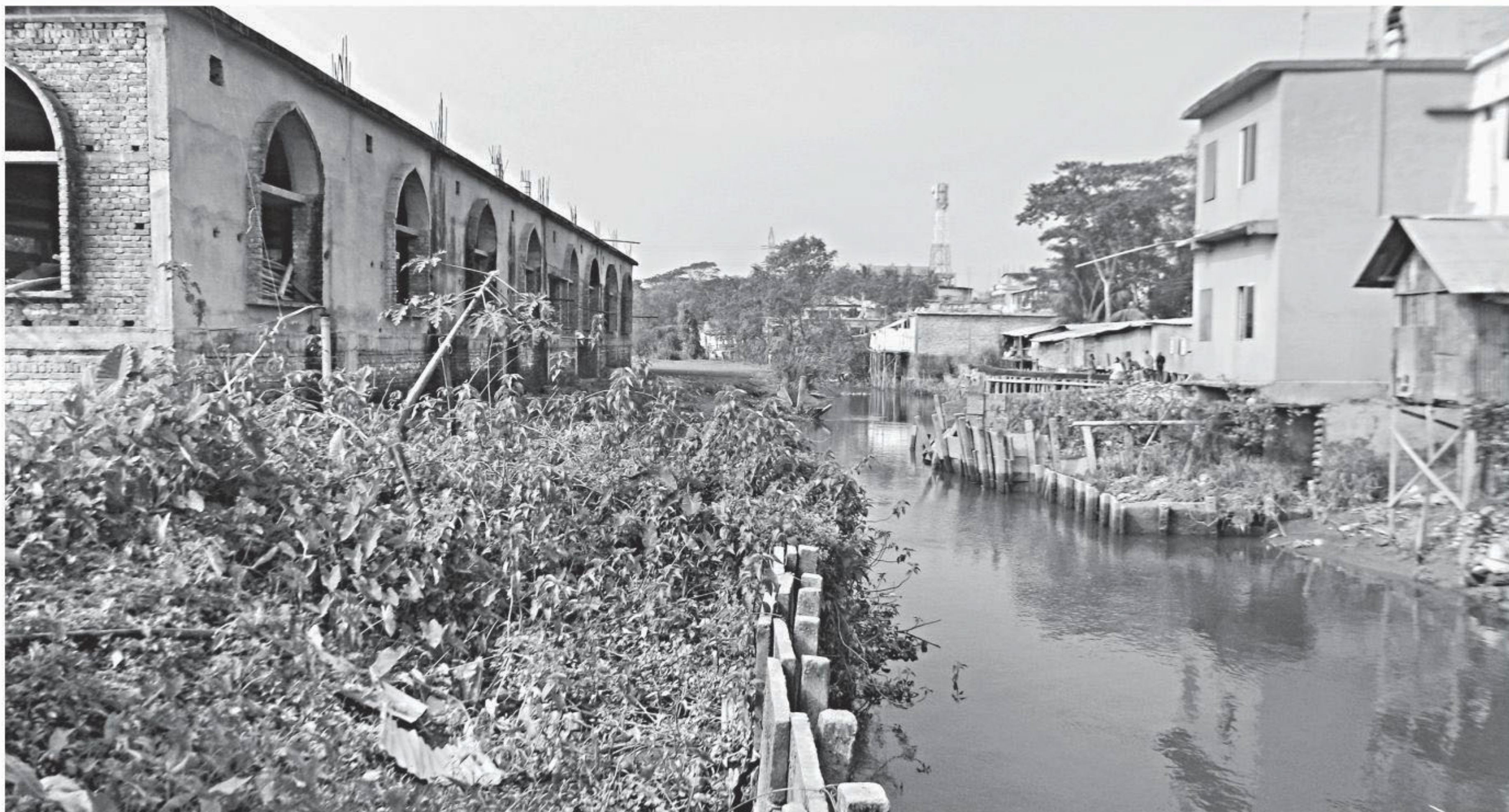
Land grabbers construct buildings at Hetalia Badghat Bazar, below, and Gorur Badghat Bazar on the Bahalgachia canal, choking the natural waterbody flowing between Patuakhali municipality and Kalikapur union in Sadar upazila of the district. The photos were taken on December 20.
