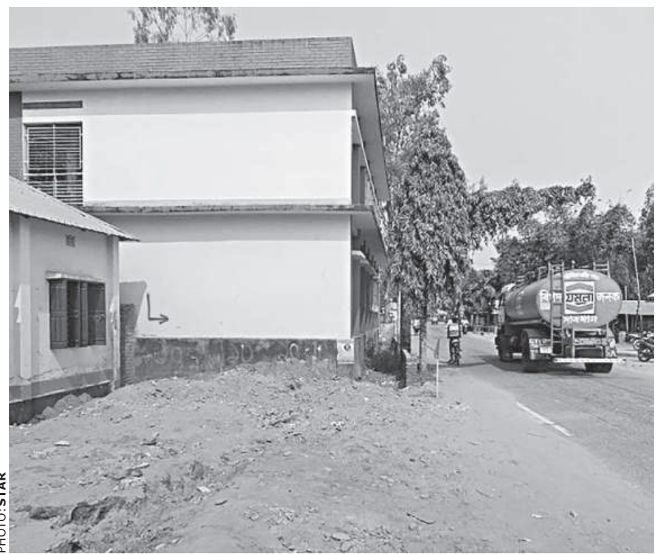
Local Government Engineering Department constructed the first floor of Dristinandan Government Primary School Nilphamari's Domar upazila in 2015 though Roads and Highways Department acquisitioned the school land (market in red arrow) in 2011.
