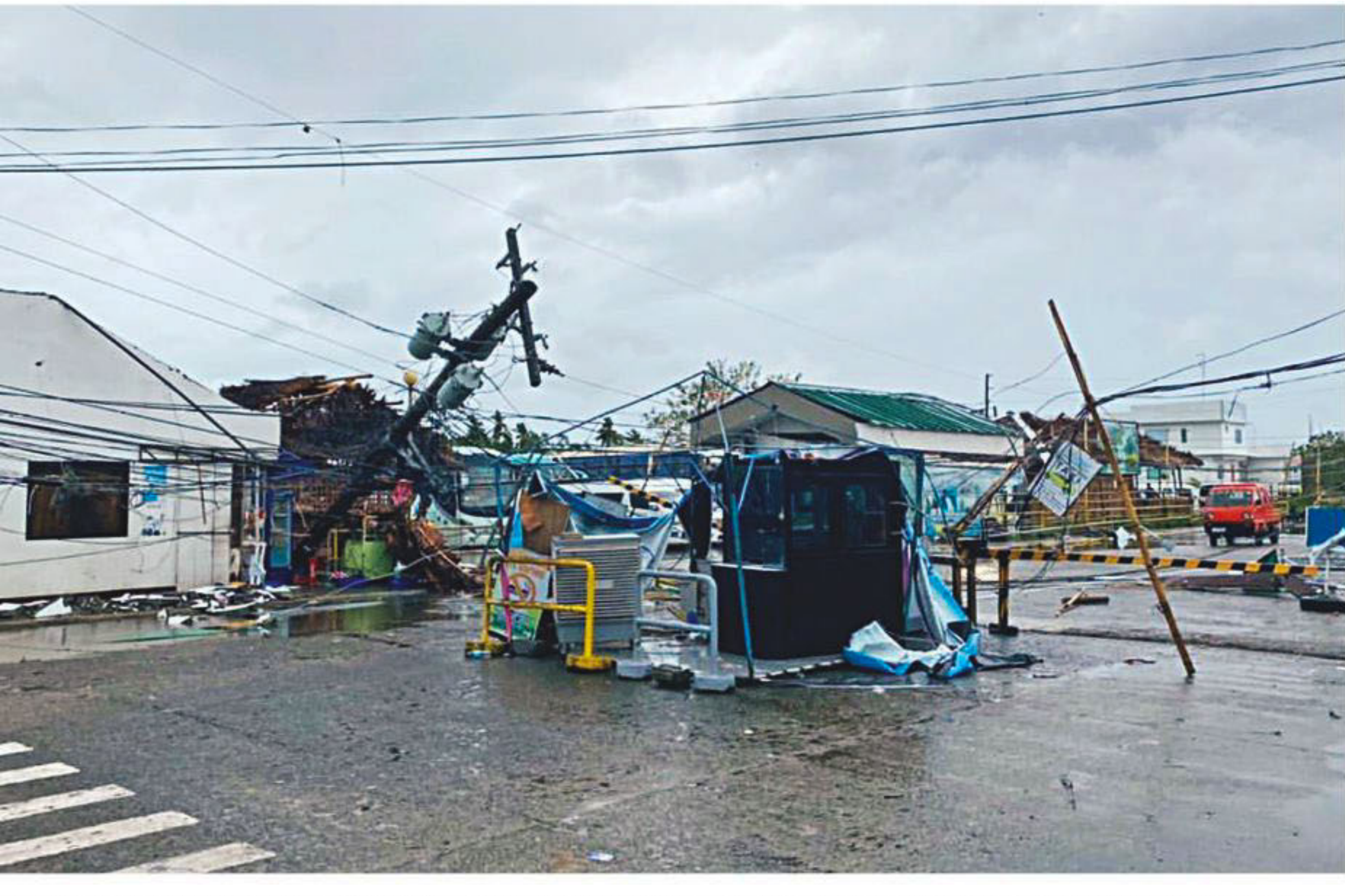
This photo shows damage to infrastructures caused by Typhoon Phanfone outside Kalibo International Airport in Kalibo, the capital of Aklan province. At least 16 people were killed in the typhoon that hit the Philippines on Christmas Day.
