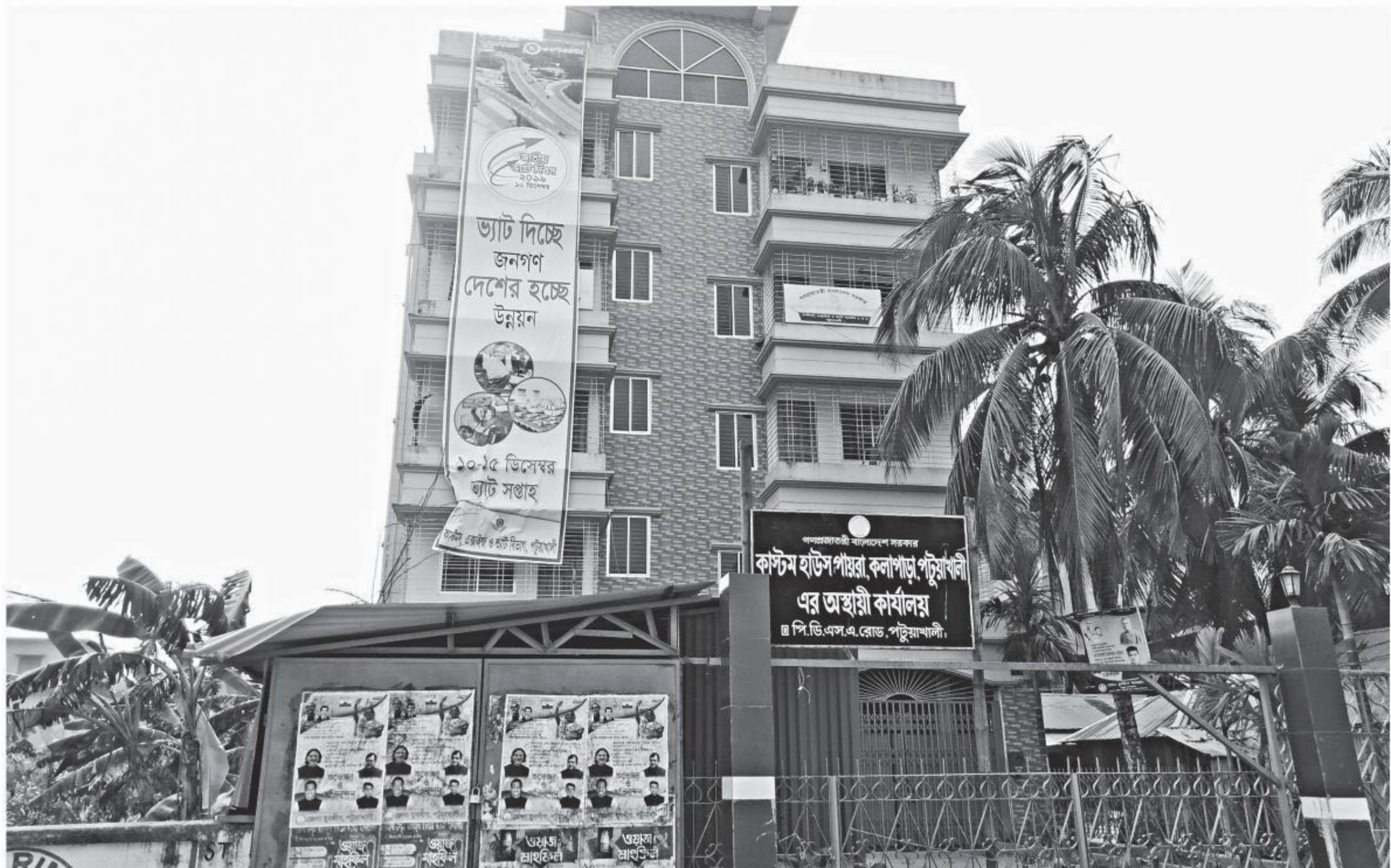
Patuakhali customs office runs its activities in this rented building in the town.
