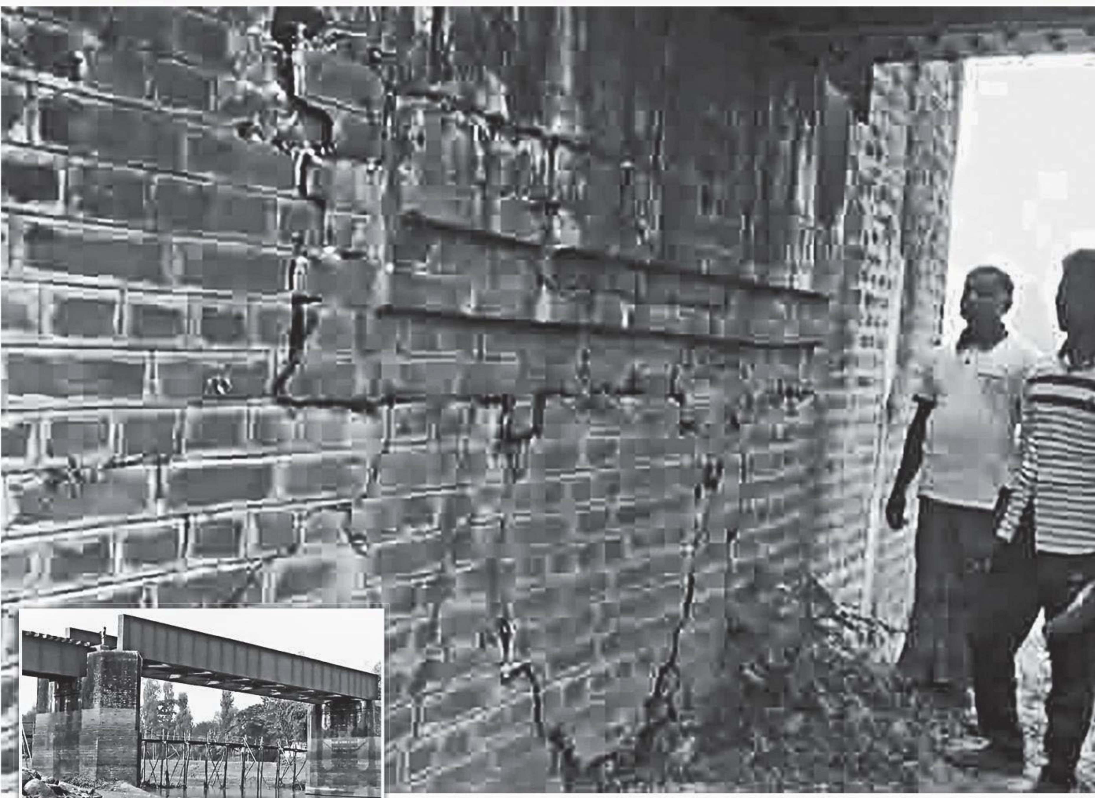
Railway workers take a look at the cracks that developed in one of the piers of the century-old Bheramara rail bridge, inset, over the Ghaghot river near Gaibandha rail station. The photo was taken recently. PHOTO: STAR
